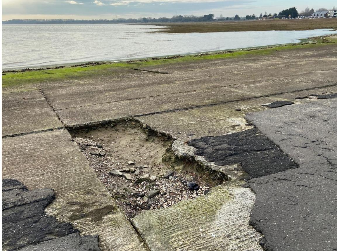
Serious deterioration of the apron with the proposed outfall in the distance.
