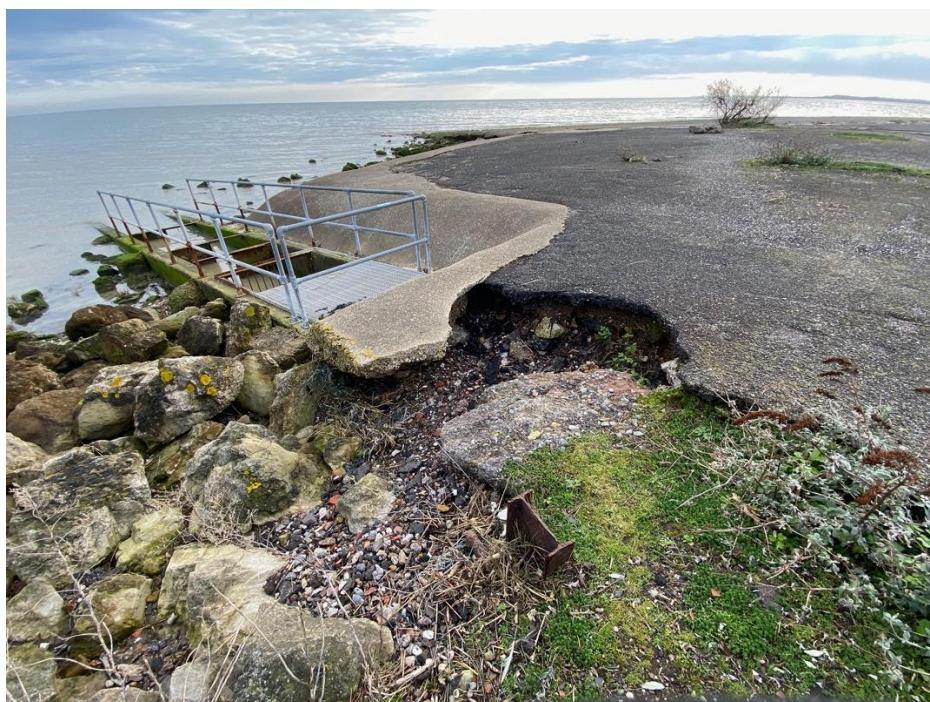
Heavy erosion next to pipe outfall exposing possible coal spoil below.
